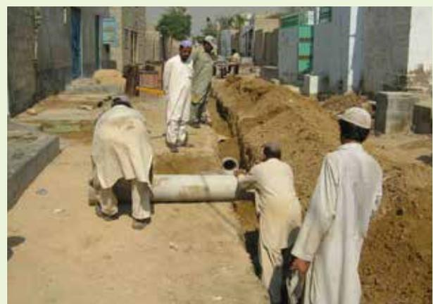
Construction of a self-help lane sewer in Gulshan-e-Zia. Street scene: during laying of sewerage pipe on self-help (background: OPP-RTI technical advisor supervises). Photo: Orangi Pilot Project.
